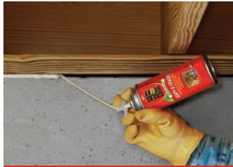
Rim joist/Sill plate
