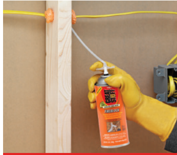
Seal Electrical Through Wall Studs
