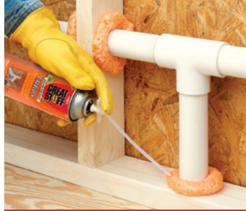
Seal pipe penetrations
