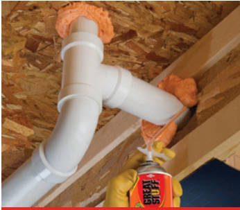
Seal pipe penetrations
